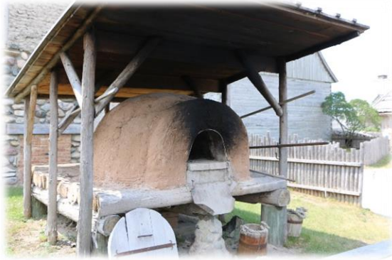
The bread oven currently sits on the location of the upcoming addition and will be moved to a more historically accurate location outside the palisade wall
